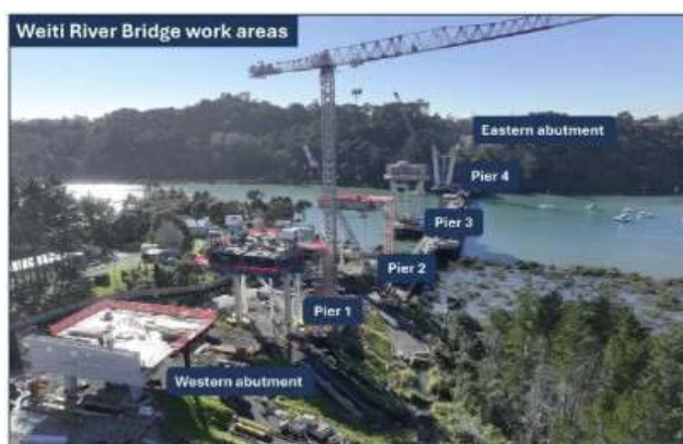
6. Penlink O Mahurangi Project – June 2026
